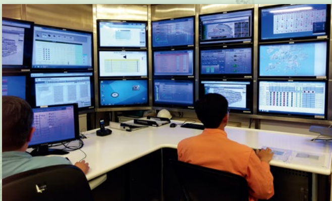
位於赤鱸角機場民航處總部的機電署控制中心，透過遠程監察系統，全天候監控八座航空障礙燈基站的運作情況，可即時找出障礙燈系統出現故障的原因。 The EMSD's control centre in the CAD Headquarters at the Chek Lap Kok Airport monitors the operation of eight OLS round the clock through the remote monitoring system to immediately identify the reasons for any failure of the obstacle light system.
