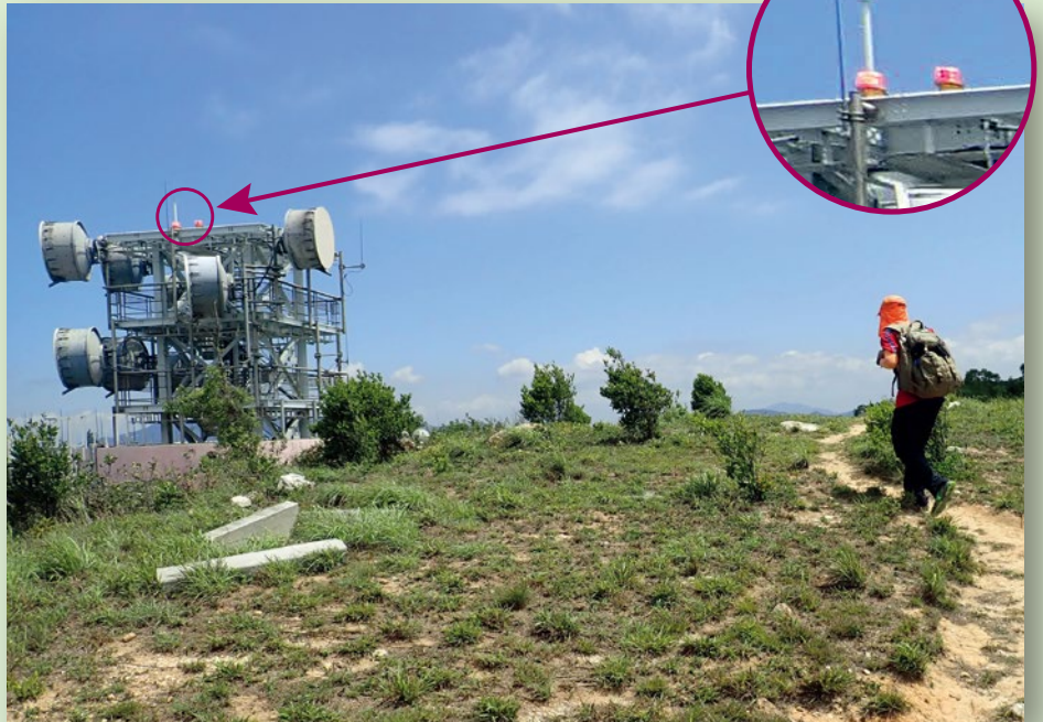
基站安裝不間斷電力供應系統後，可減少前線工作人員進行緊急維修的次數。小圖為航空障礙燈。 The installation of UPS system at the station can reduce the frequency of frontline staff conducting emergency repair. Shown in the circled picture is the obstacle lights.
