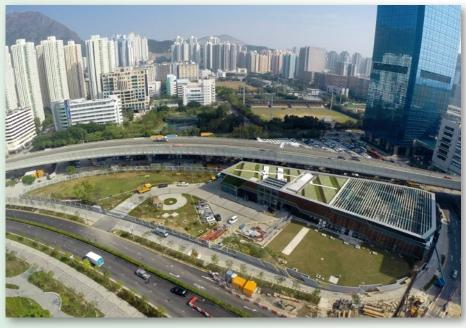
區域供冷系統的能源效益較傳統風冷式空調系統高約35%,亦較使用獨立冷卻塔的水冷式空調系統高約20%。 The energy efficiency of the district cooling system is about 35% higher than that of the conventional air-cooled air-conditioning system, and about 20% higher than that of the water-cooled air-conditioning system which uses separate cooling towers.
