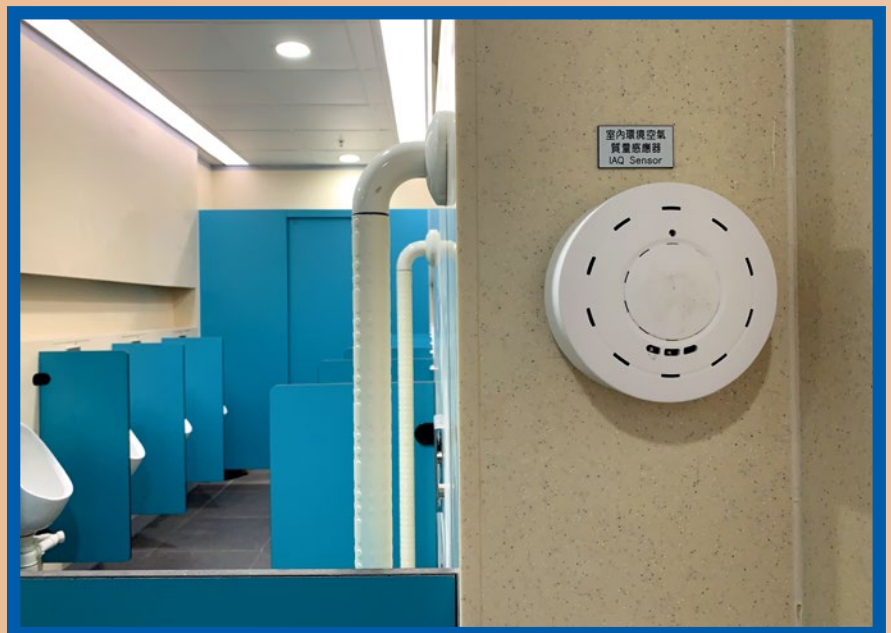
安裝在智能洗手間的室內環境空氣質素感測器。 Indoor air quality sensor installed in a smart washroom.
